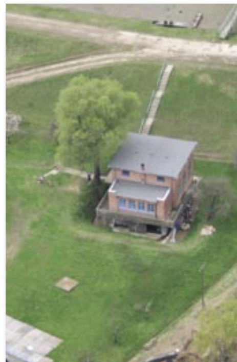
Pump station behind dyke
