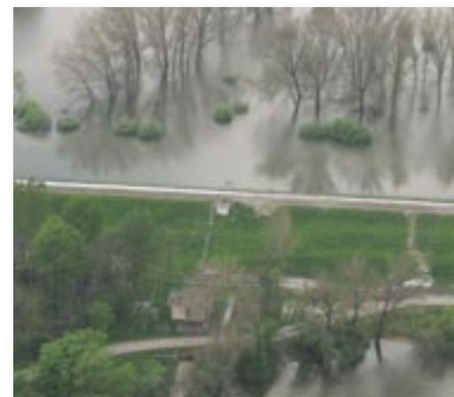
Pumping plant below the water level and behind sandbags
